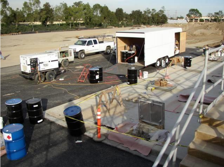
Figure 9: Typical field staging and setup
