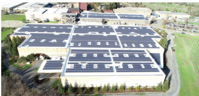
SPF roof with photovoltaic panels at the Rodney Strong Vineyards in Healdsburg, CA.
