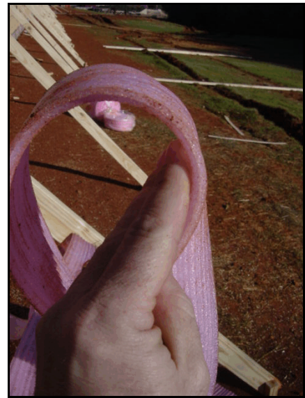
Figure 14. New sill sealer.
